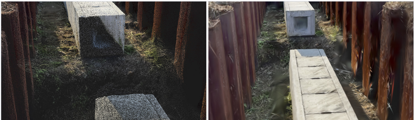
Check the geometry, not the render: the same trench as point cloud (left) and 3DGS scene (right)
